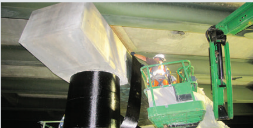
Application of RenewWrap FRP around column for confinement.
