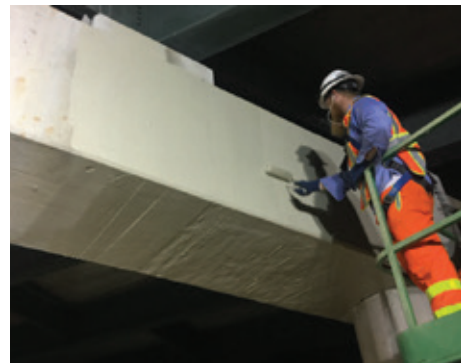
Painting RenewWrap FRP system with epoxy coating.
