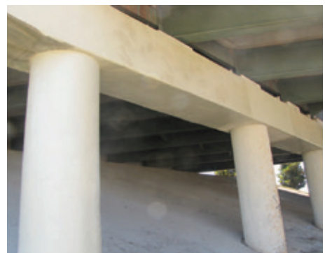
Completed column and pier cap.
