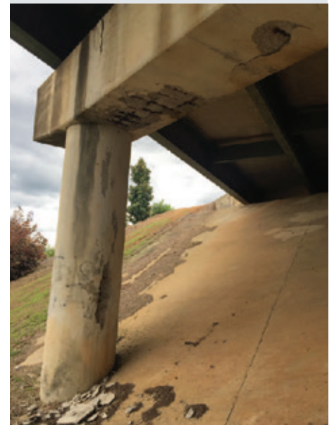
Column and pier cap prior to repair.
