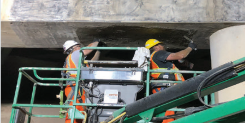
Application of GeoStrong repair mortar.
