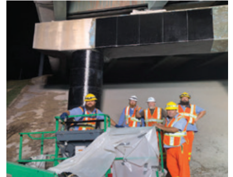
Completed repairs prior to coating.
