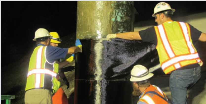
SCDOT maintenance crew wrapping pier cap with RenewWrap FRP system.
