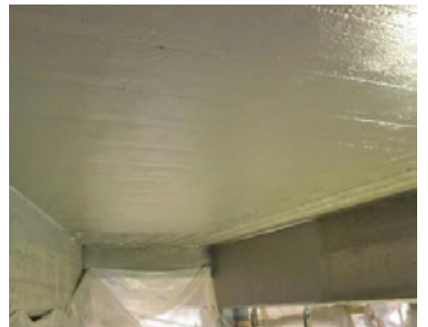
Completed deck strengthening after coating with UV-resistant paint
