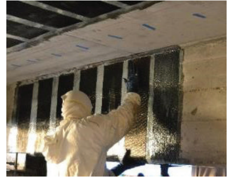
RenewWrap carbon fiber U-wraps used to increase shear capacity of floor beams
