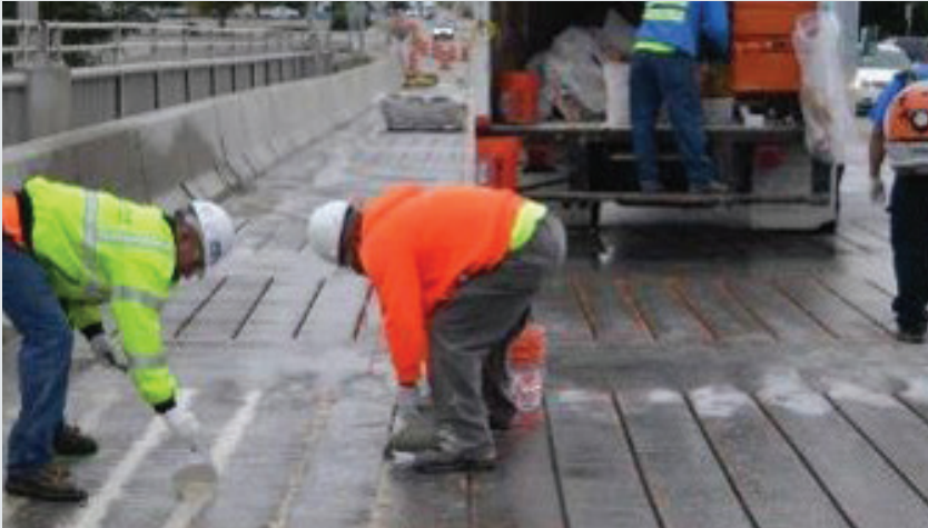
Installing CFRP bars in slots for negative moment strengthening
