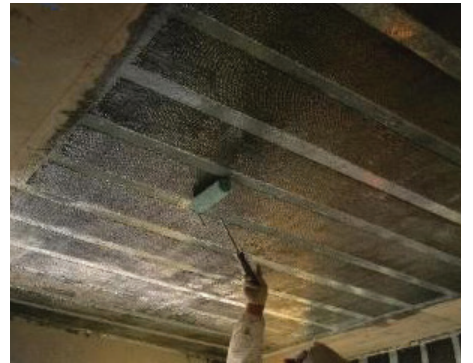
RenewWrap carbon fiber bonded to deck soffit to increase positive moment capacity
