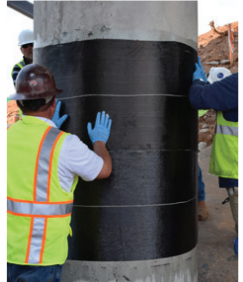
The crew wraps the column under the intersection of I-85/I-385 in South Carolina
