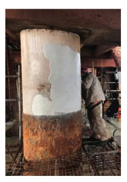
Figure 2: Epoxy putty installation process.
