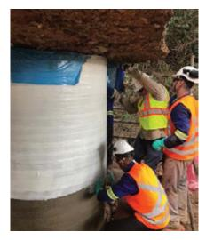
Figure 5: Application of two Syntho-Glass XT layers.
