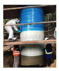
Figure 6: Application of compression film on top of the Syntho-Glass XT layers.
