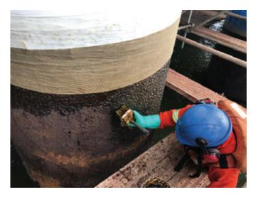
Figure 8: Staggered system layers on a repaired section and beginning of the installation of the next repair section.
