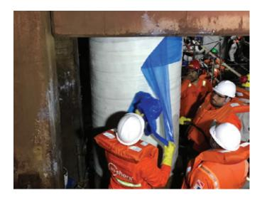
Figure 7: Removal of the compression film and installation of the Syntho-Glass SPF.
